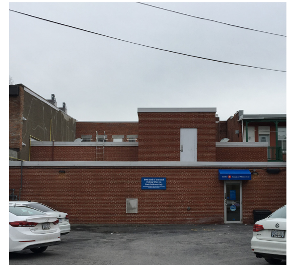
Rear Elevation of 159 Pitt Street. Photo by +VG Architects, 2018.
