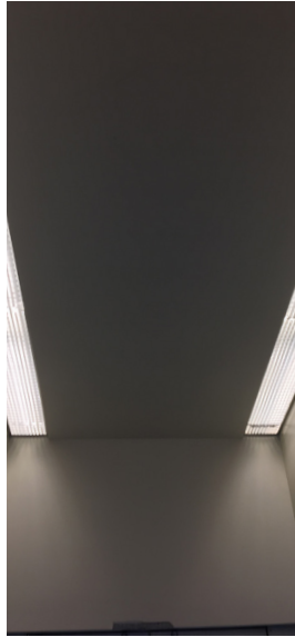
Interior ceiling and lighting conditions.
